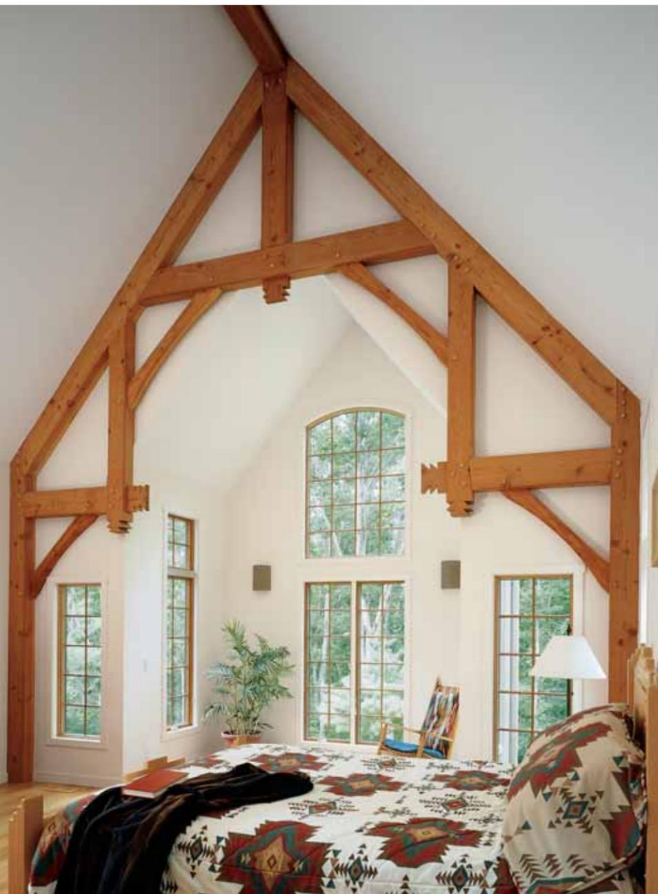
**ABOVE:** In keeping the home's Southwestern decor, the framing crew hand-cut the through-tenons into a jagged shape, which resembles the pattern of the comforter in the master bedroom.
